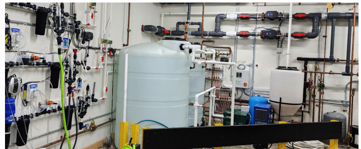
The Lotus nanobubble generator is installed on the grow day tank.
